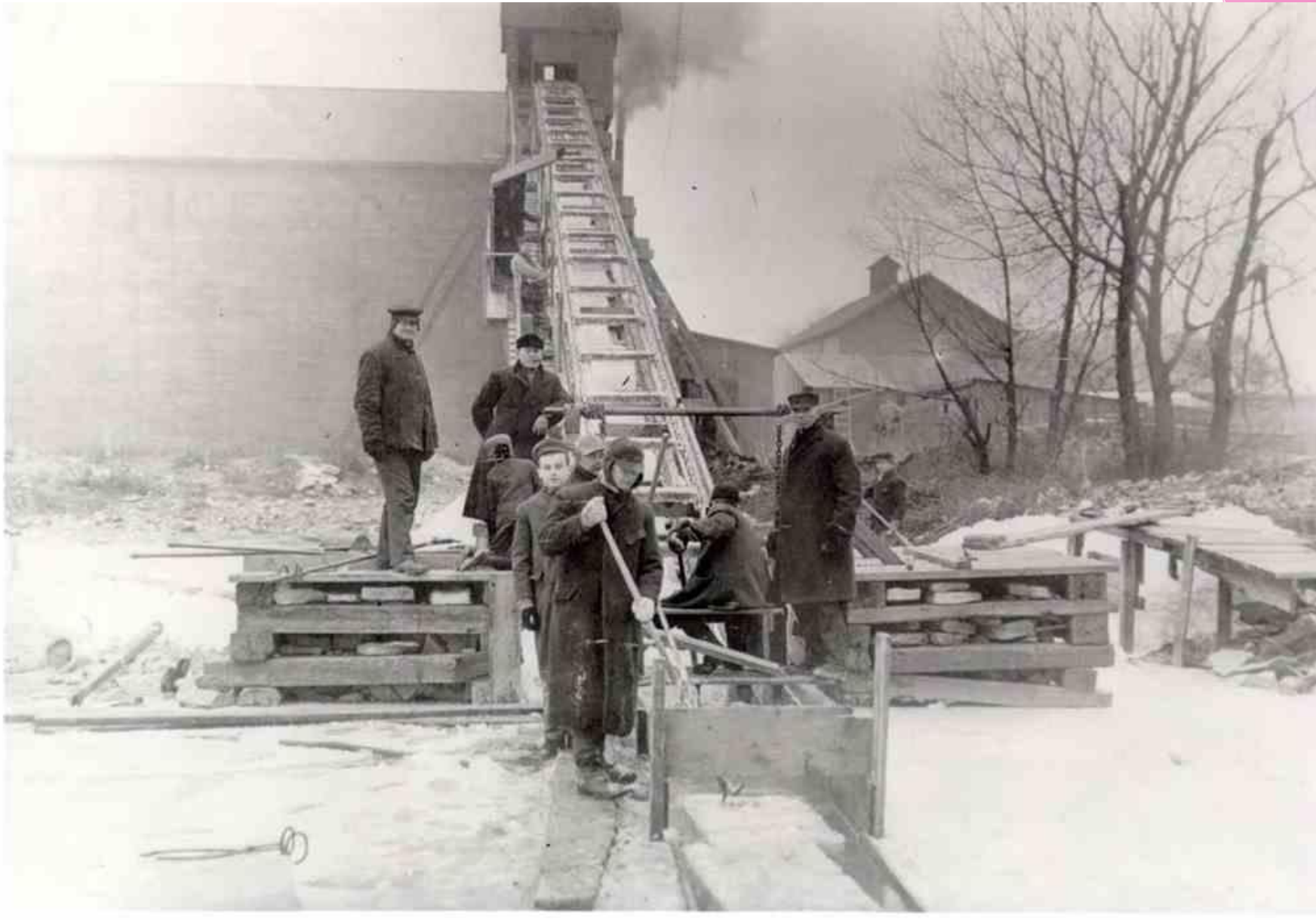
Conveyor belt used to move ice blocks from pond to ice house. Sandusky Bay (OH) off Lake Erie.
